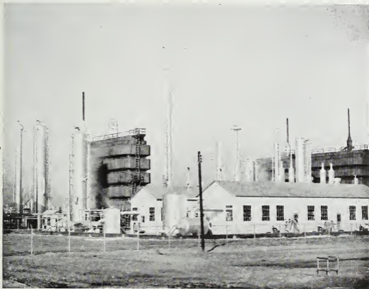
Natural gas plant at Lake Centralia, Illinois.
